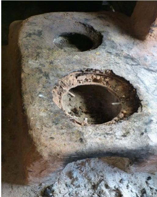
Figure 7: IICS in police barrack with damaged pothole
